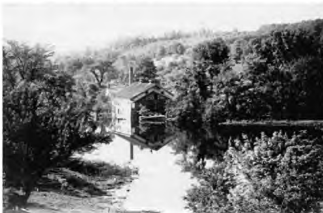
A southerly view of the Crosby and Robinson paper mill, showing the large containment of the Konkapot River's water above the mill dam.
