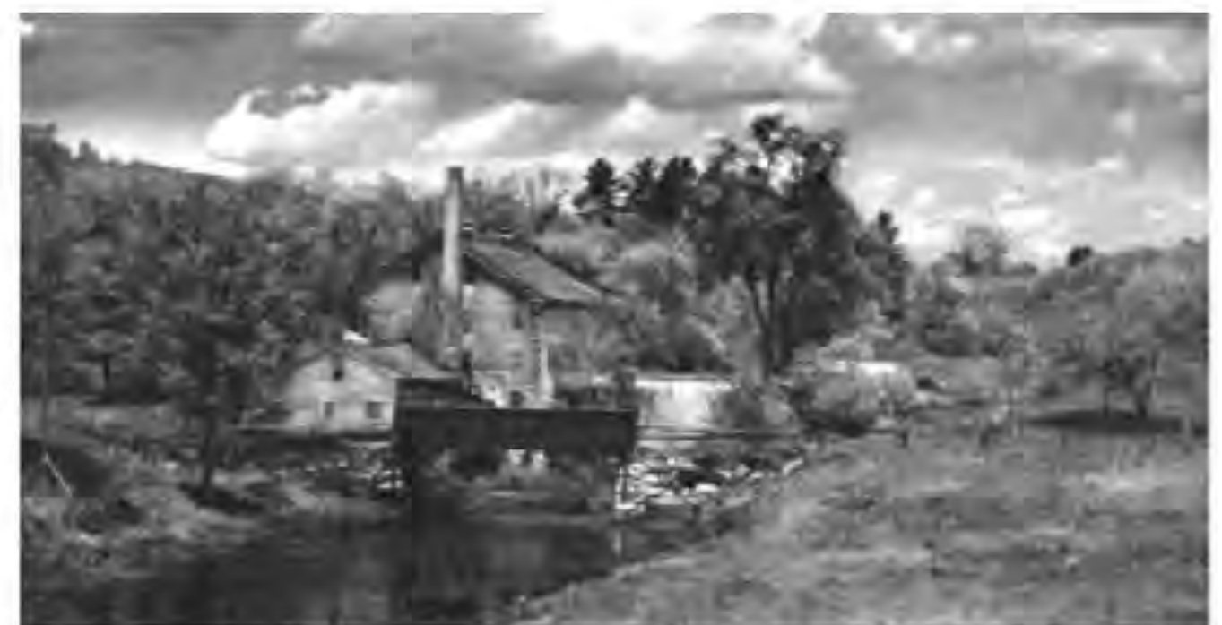
A late nineteenth century photograph of the Crosby and Robinson paper mill. The dam that supplied the power for this mill, located just north of the Hayes Hill Road bridge, was largely destroyed in 2012 by Hurricane Sandy's heavy rains. The impressive foundation of this mill still stands, and is well worth a visit.
