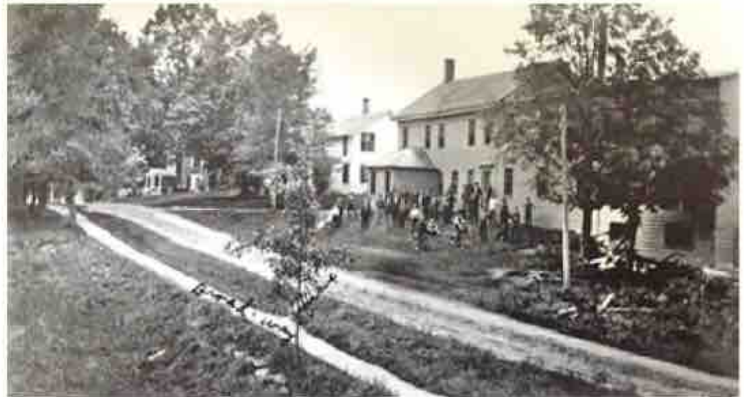
Upper right, the present-day Whip Shop and (right) the building in 1908, which some wag placed at the intersection of Broadway and Fifth
