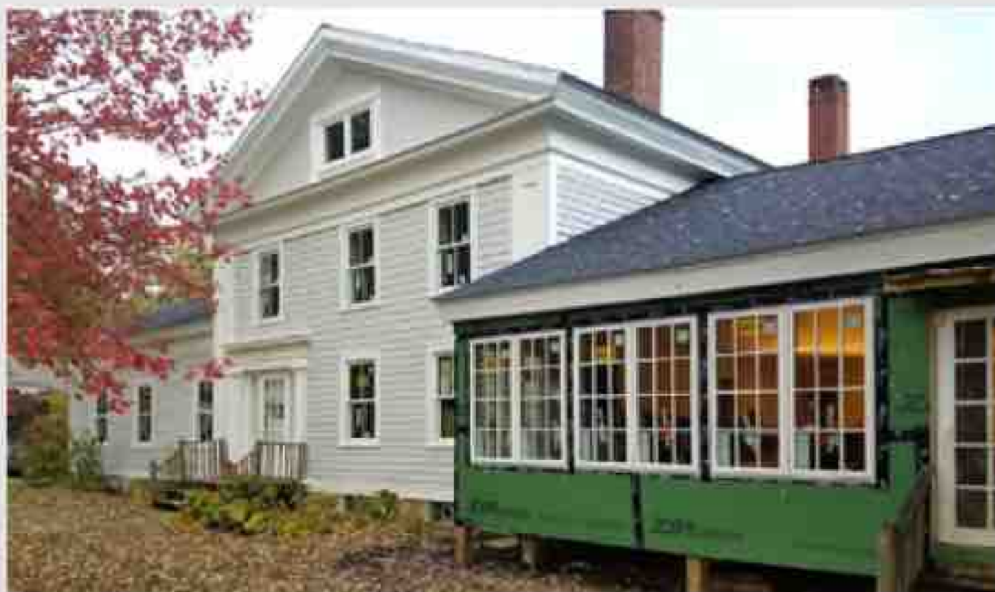
Mill River Village House with renovations well under way
