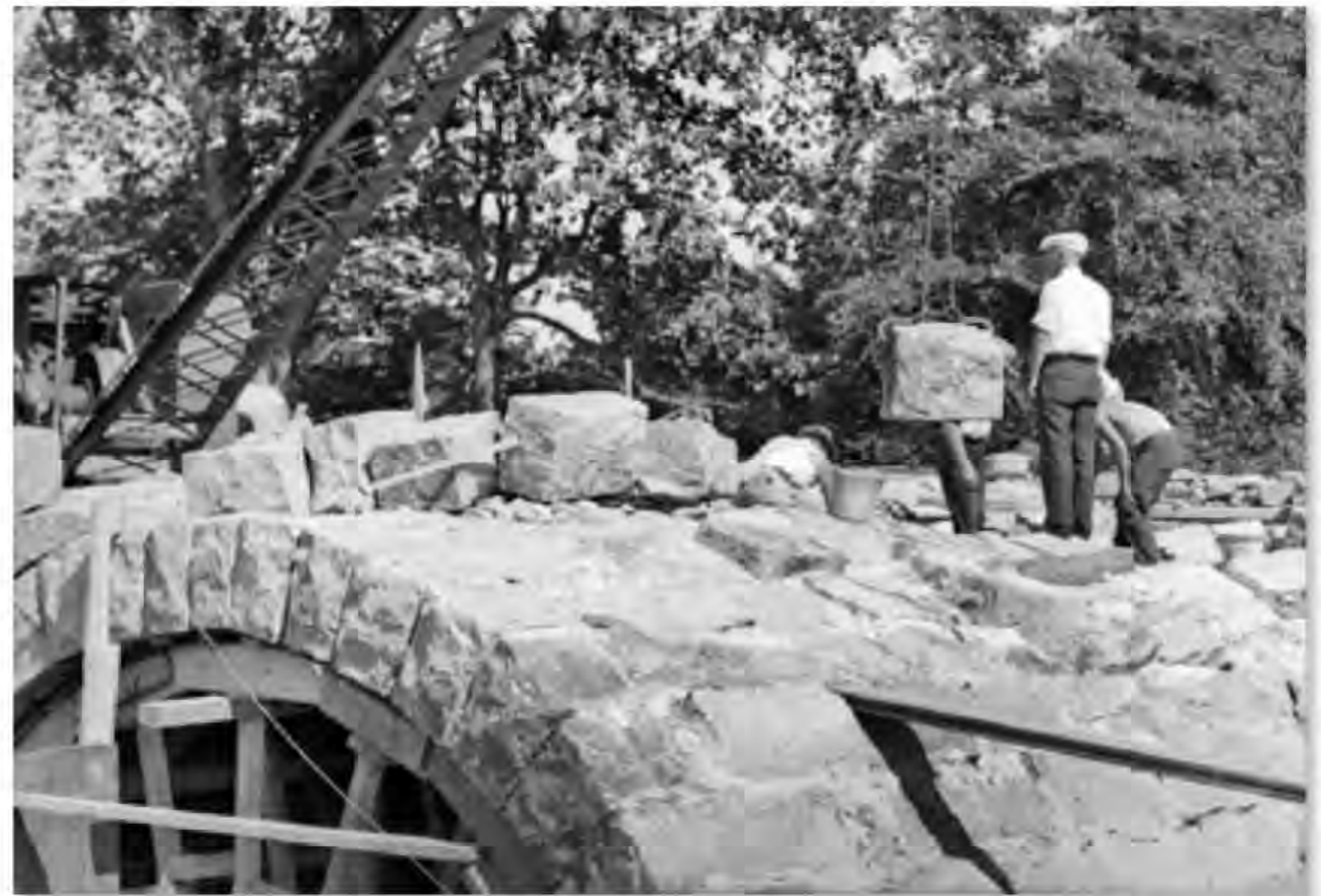
A keystone bridge under construction in the early part of the 20th Century.
