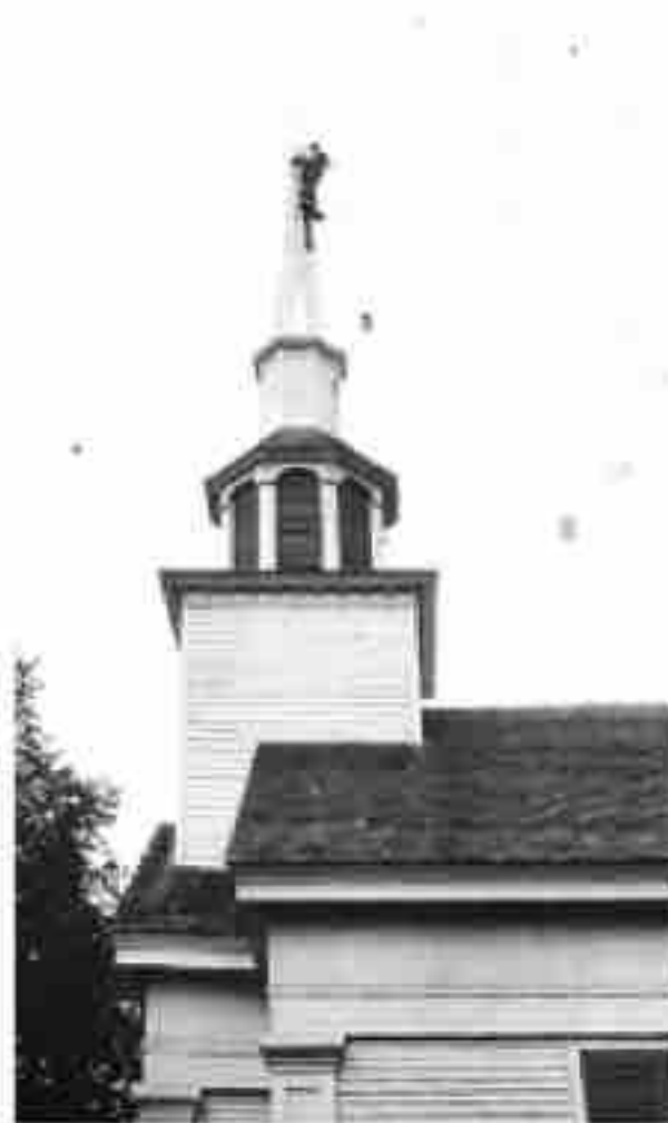
Left, painting the steeple in 1926 required ropes, a hook, and nerves of steel. The modern paint job, right, employed two workers: one at the controls and the other tucked comfortably into the cab of a motorized lift. photo at right by Janice Boult
