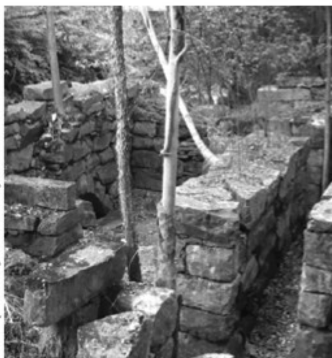
Site clearing continues to reveal the ruins of the Crosby and Robbins Mill on the Konkapot River.
