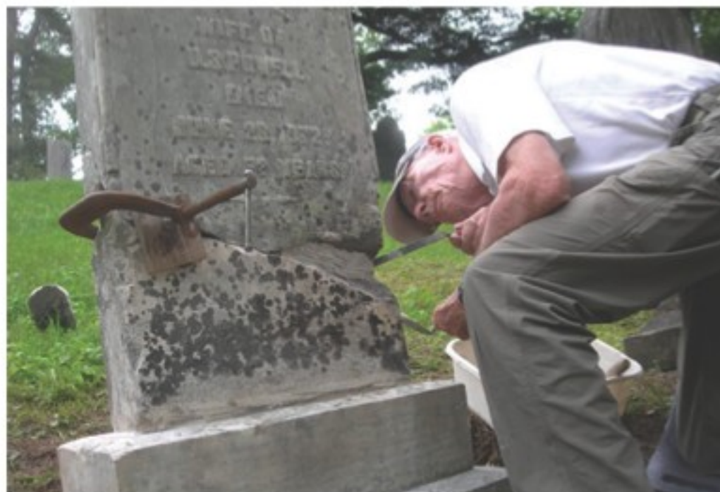
Conservator Jim Fannin repairs a broken stone with dowels, glue, and mortar.
