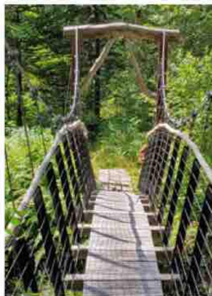
Destination: the Land Trust Bridge at the east end of Thousand Acre Swamp
