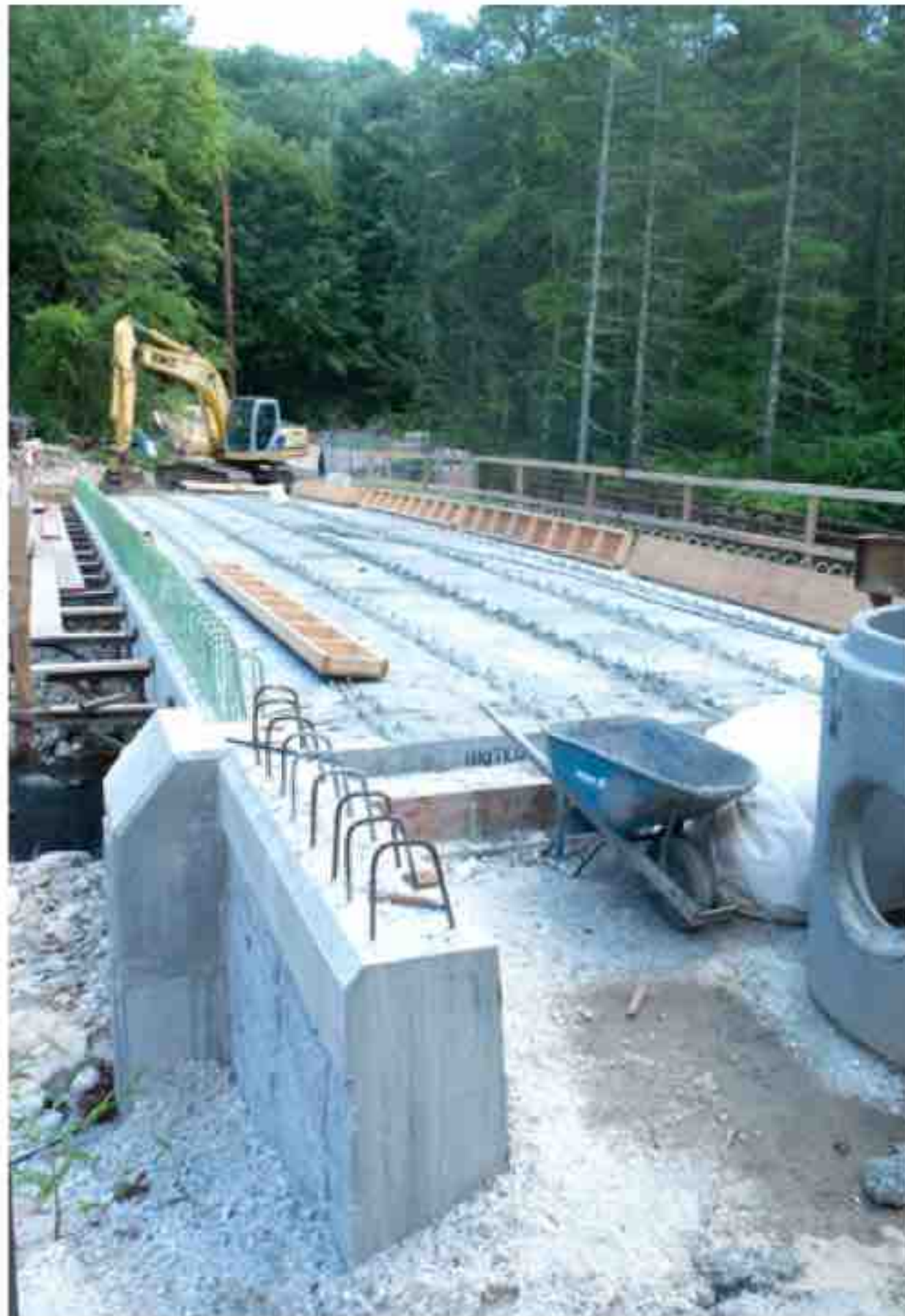
And preparing for surfacing in mid-August
