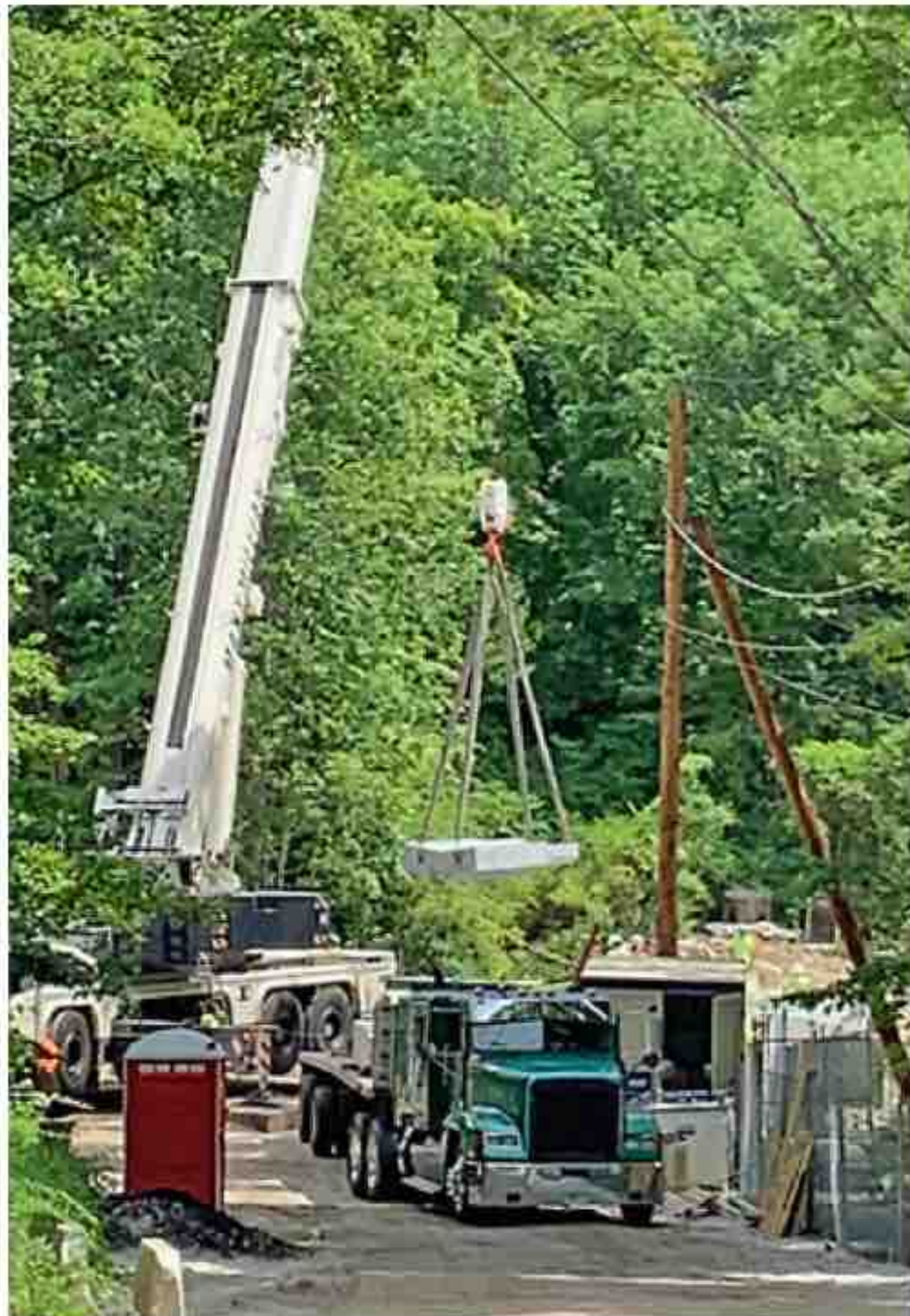
Moving concrete slabs into place...
