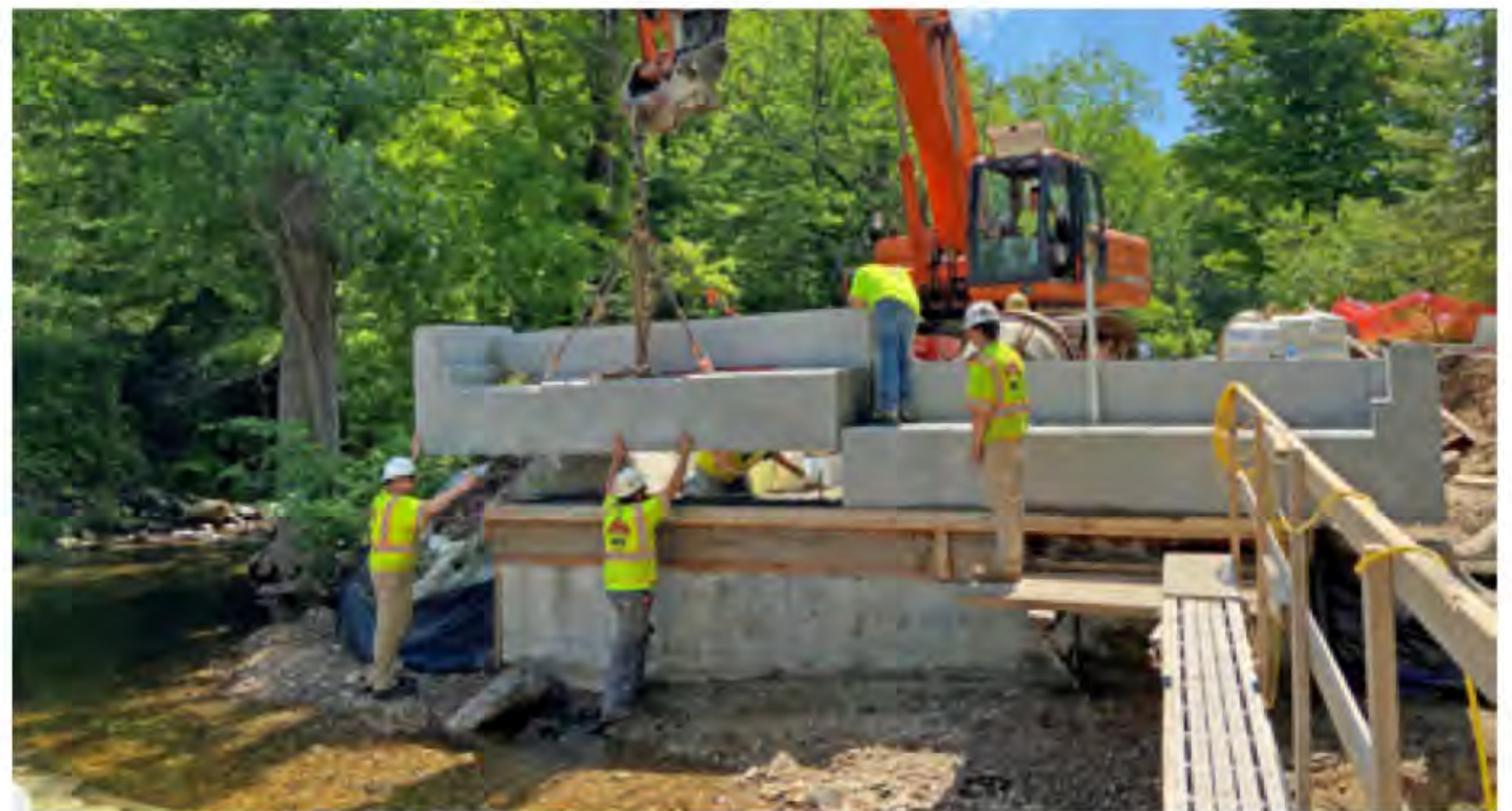
Lumbert Cross Road Progress Report: The crew converting the failing Lumbert Cross Road bridge from a single to a two-lane crossing is employing a recently instituted accelerated construction process. Highway Superintendent Chuck Loring took the earlier photo, showing the demolition of the original bridge, at the beginning of June. Just ten days later, Mr. Loring photographed the crew as it set pre-cast supports in place. At this writing, Lumbert Cross Road was still scheduled for closure until September.
