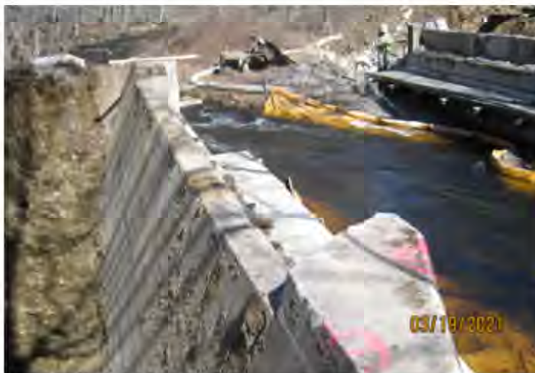
Rebuilding the Campbell Falls Road bridge
