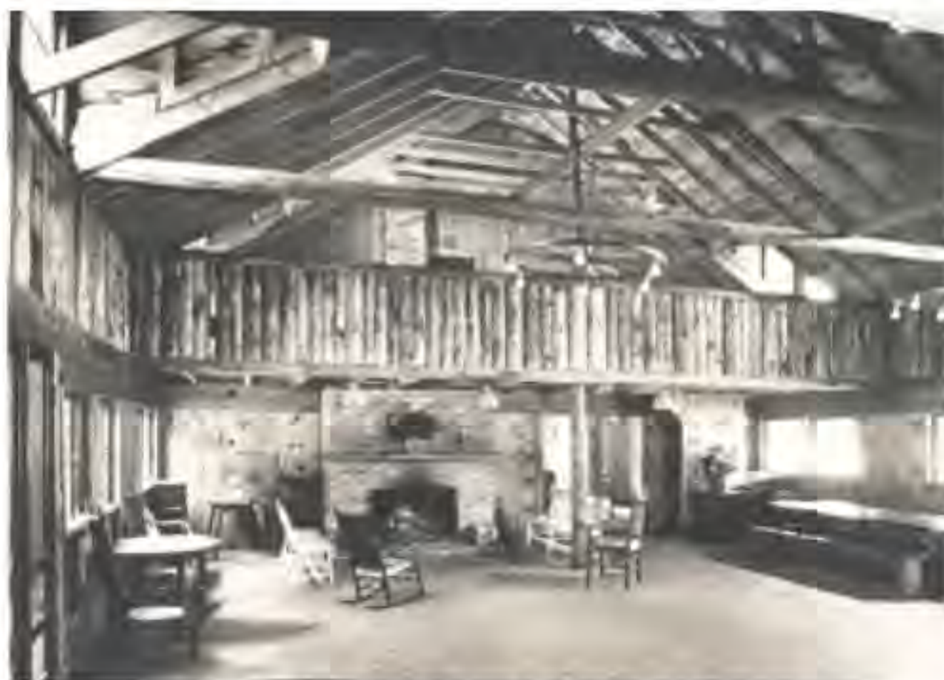
The interior of the main lodge at To-Ho-Ne Guest Camp
