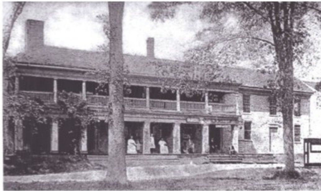
The Inn with general store and post office, late 1800s. Photo from New Marlborough Historical Society archives
