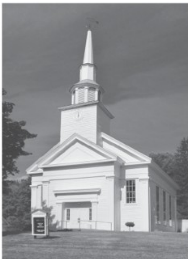
The Southfield Church
