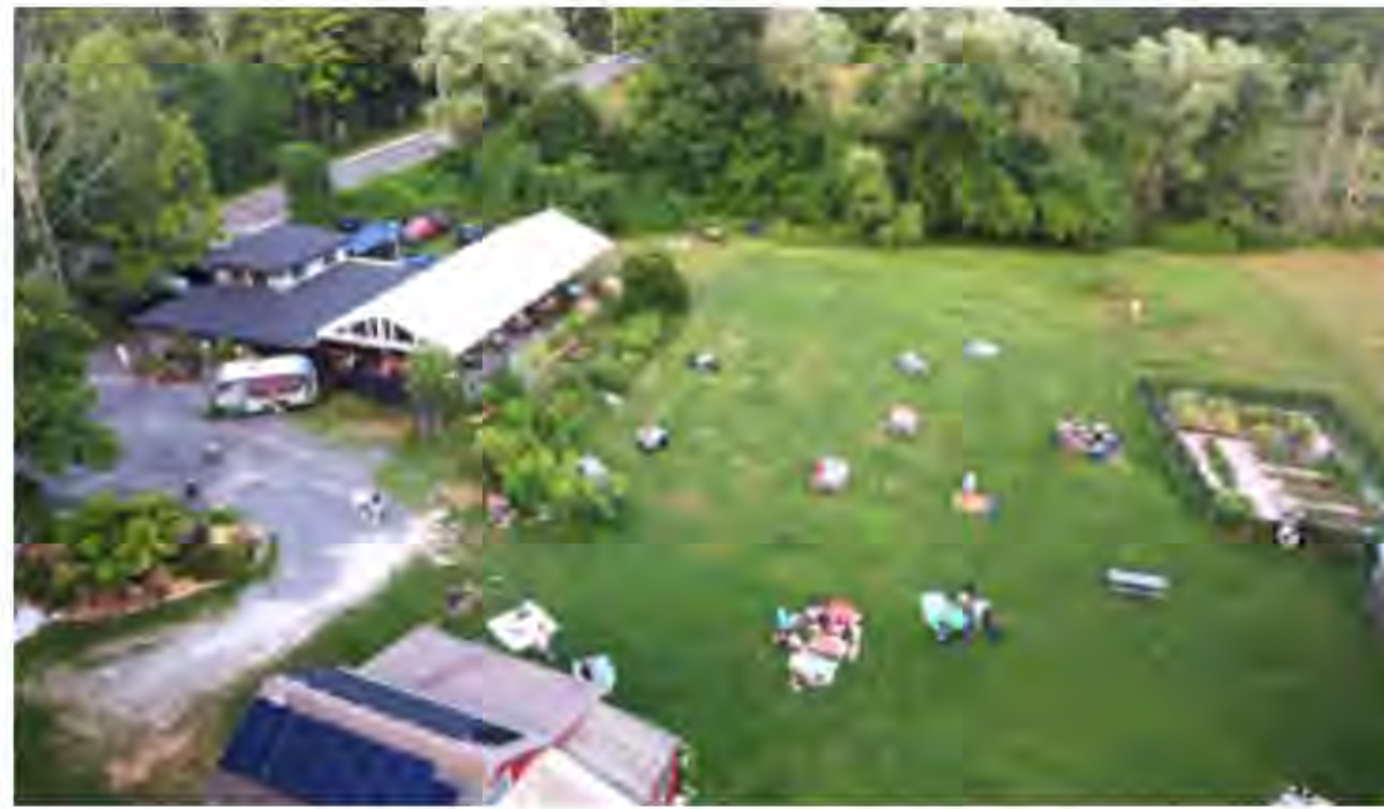
Aerial view of the Cantina 229 restaurant
