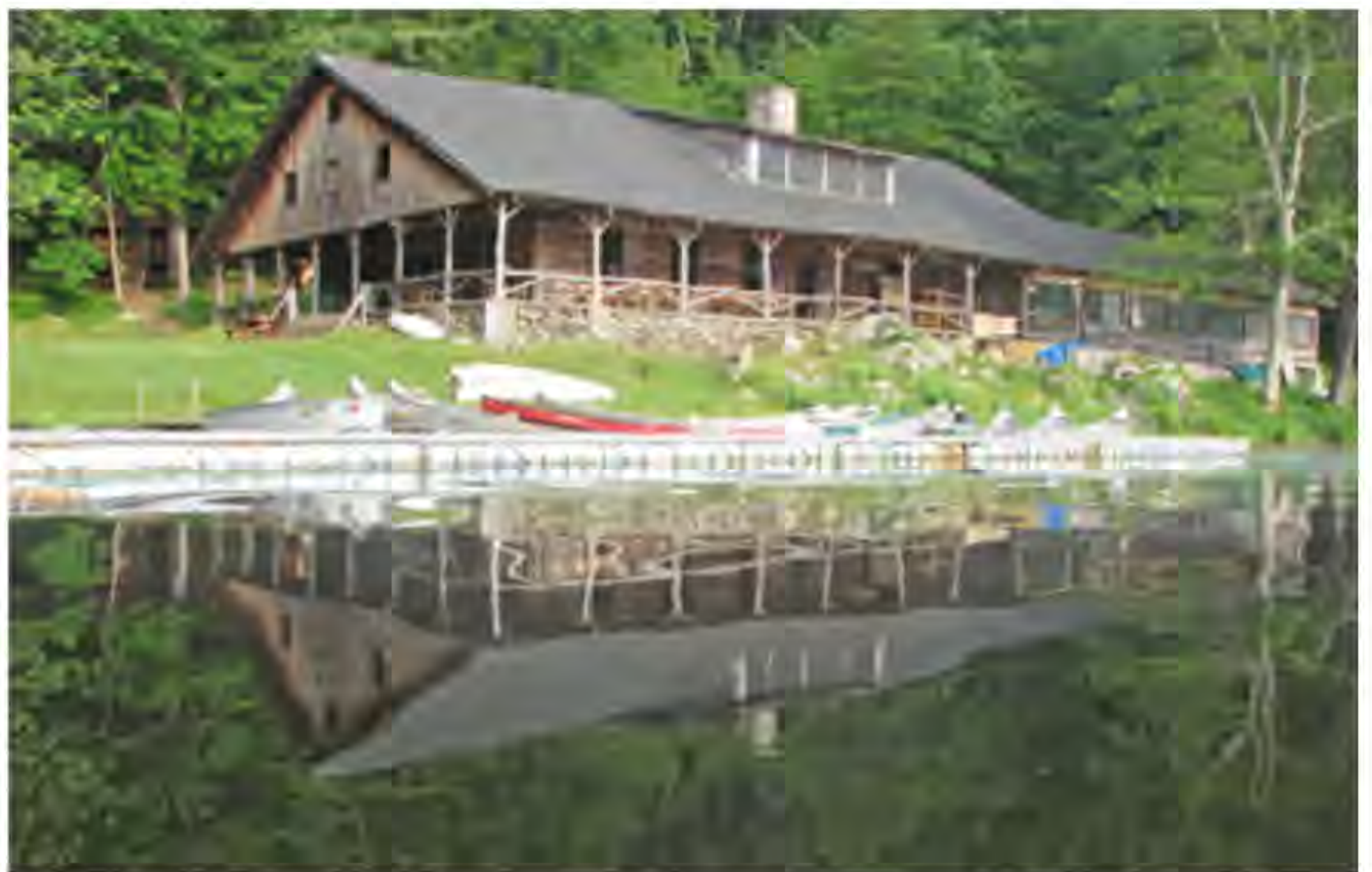
The Wa Wa Segowea lodge, built on the banks of Harmon Pond, is slated for renovation.
