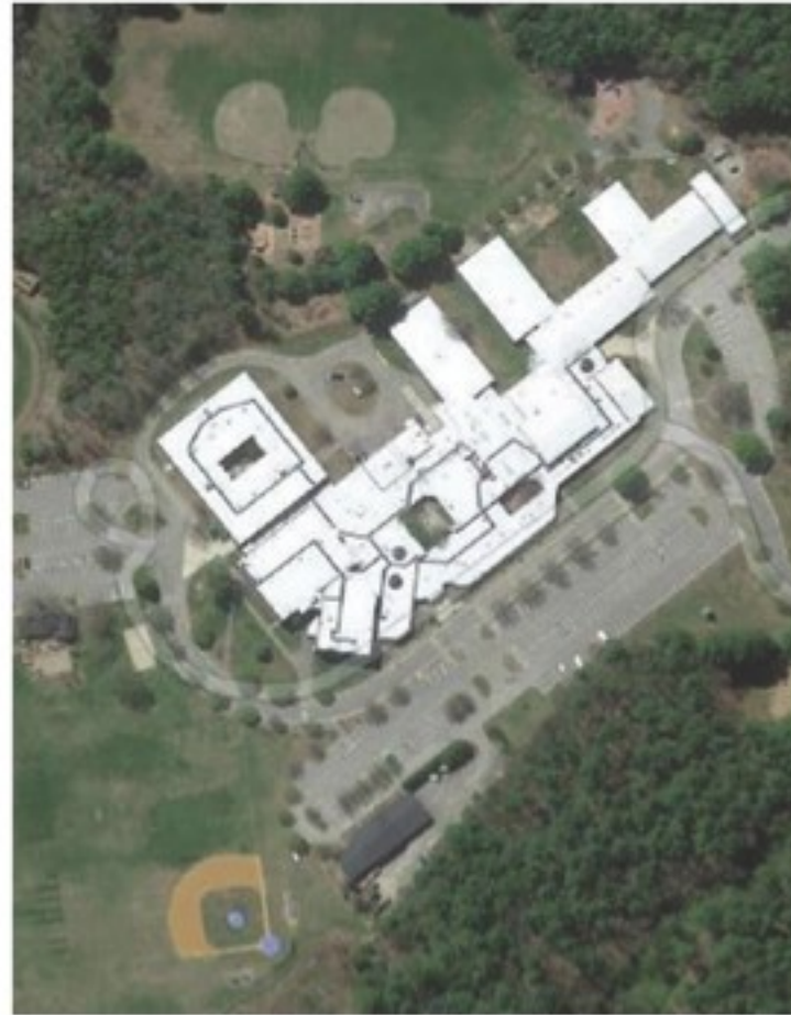
The Mount Everett High School roof spans four and a quarter acres.
