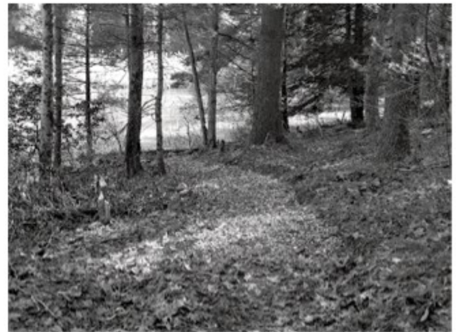
The trail under construction at the Joffe Project
