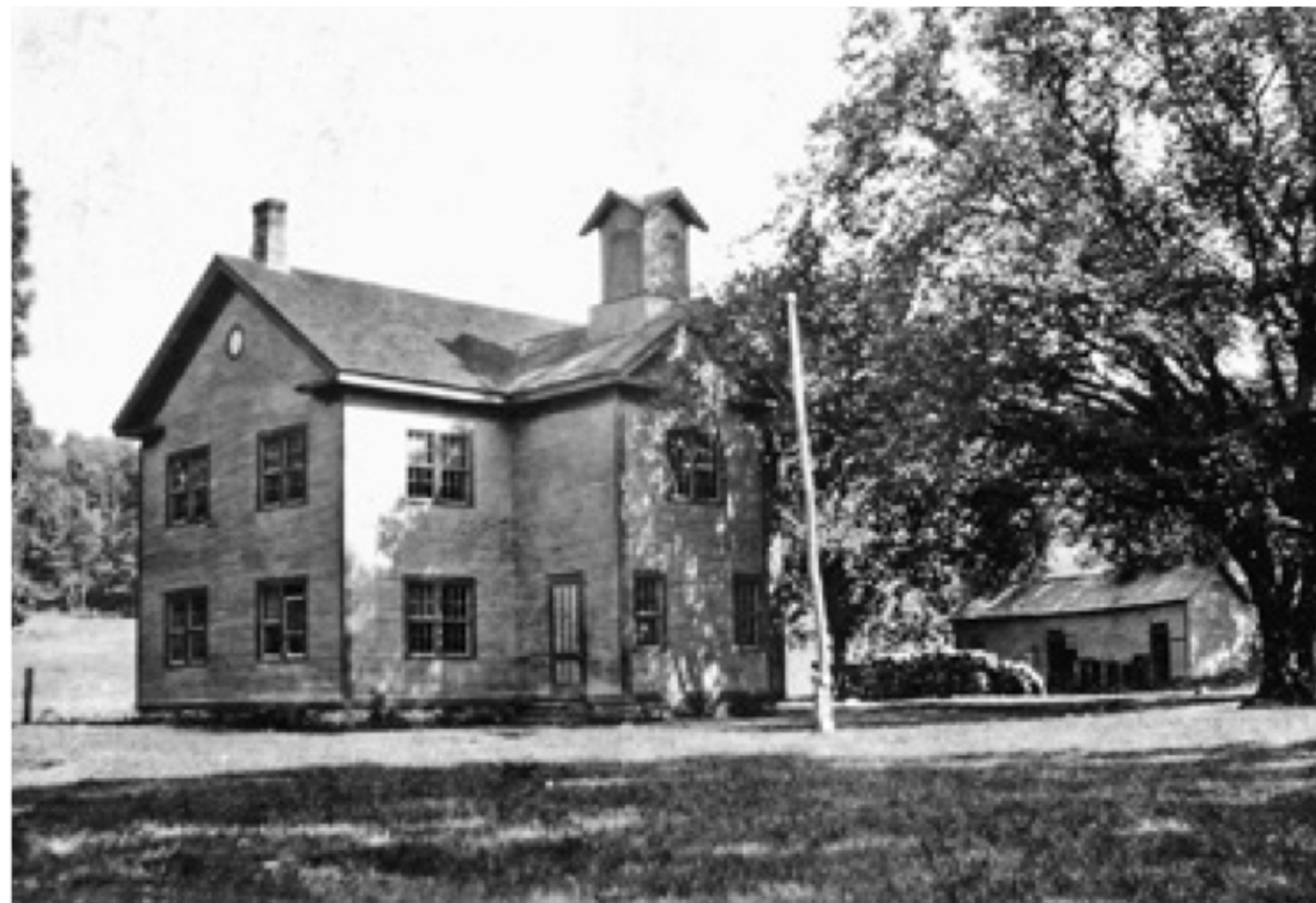
The former New Marlborough School in Mill River, which was torn down in 1932 to make way for the brick building, now known as New Marlborough Central School.
